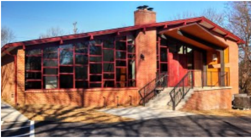
Completed exterior rebuild-the new wall of glass – photo credit Jake Short
